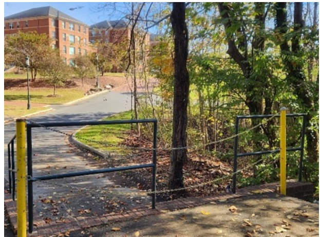
Trash Dumpster Platform With Guardrails
