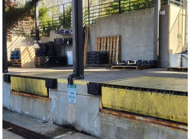
Loading Dock with Dock Plates
